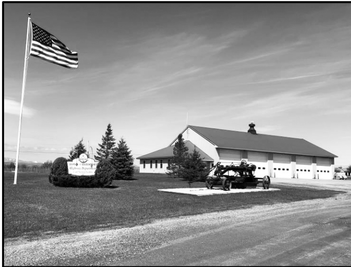
Town Garage in April 2020.
